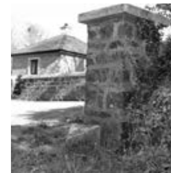
Fig. 15 (R.): Aghills, entrance to Shepperton Estate located between Leap and Skibbereen (Photo: author). 41
